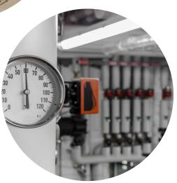
Monitor the temperature in a water circuit Sanitary Hot Water (DHW) to avoid the multiplication of bacteria called Legionella causing legionellosis.
