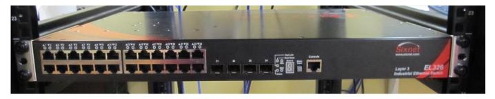
The above image shows an EL326 in front style arrangement (ports in front and power in the back) mounted in a typical 19" rack, prior to wiring.
